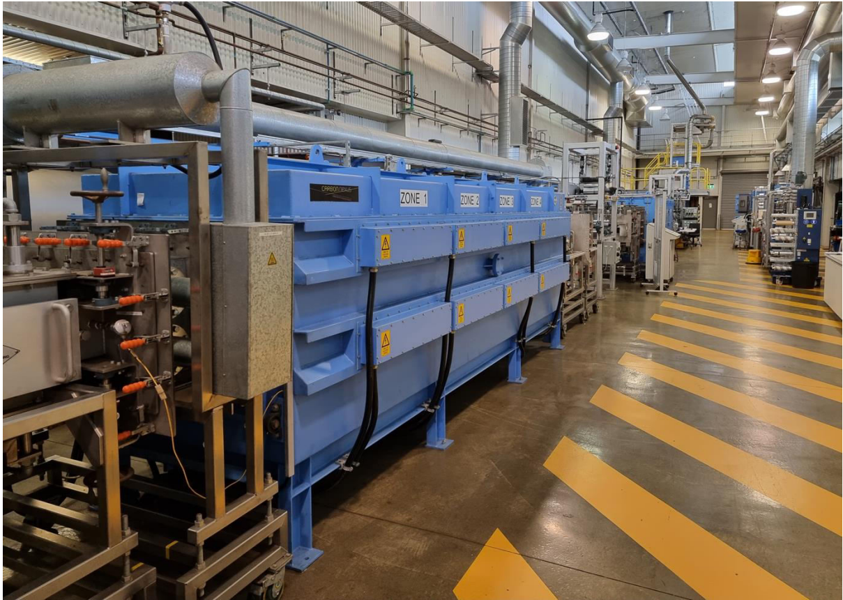
Industrial scale machinery for the production of carbon fibres
